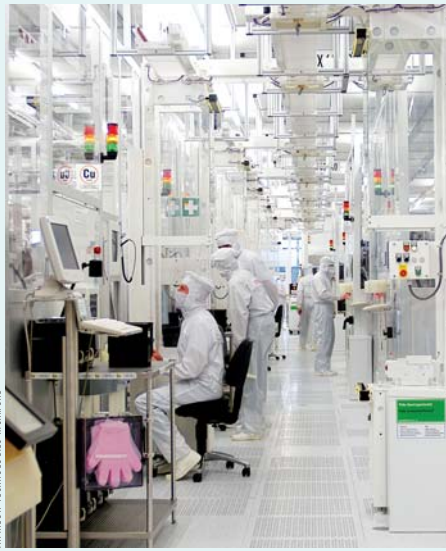
Virginia's big semiconductor catch turned out to be Infineon Technologies. The company built this clean room and fabrication plant east of Richmond.
