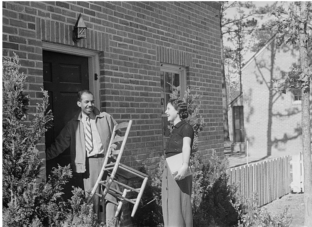
A couple moves into a new home in Aberdeen Gardens in Newport News, Va., in 1937. Aberdeen Gardens was built as part of a New Deal housing program during the Great Depression.
